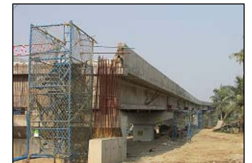
Construction of Chandernagore Flyover
